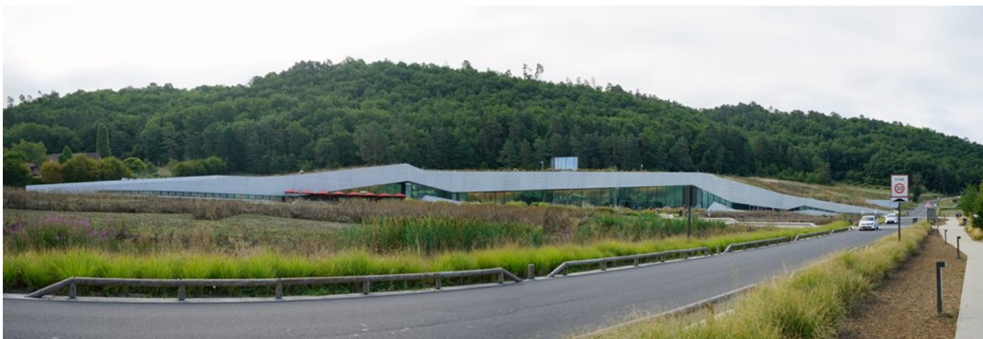
The building complex housing the International Centre for Cave Art, including the most complete facsimile yet of Lascaux Cave, Lascaux IV
